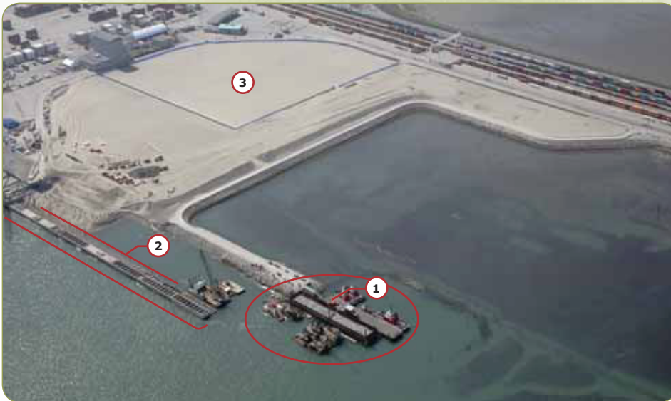
1) Tug basin, home to Seaspan's tug operations and Roberts Bank Lifeboat 2) New berth face 3) Terminal area for container storage.
